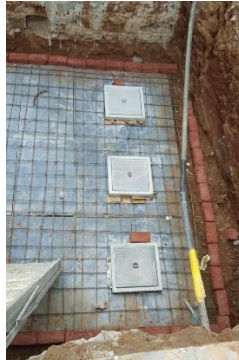
Day 8 Settling tank slab and manholes
