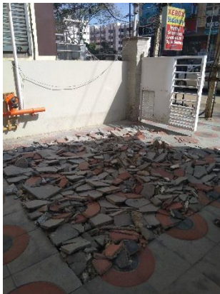
Day 1 Breaking of existing tiles and 250 mm PCC bed
