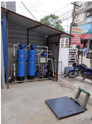
Original WTP setup with AMF, ACF, bag filter and UF. Current WTP setup with ozonator, bag filter, AMF, ACF and MCF.
