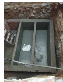
Day 6 Plastering and waterproofing on the outside and inside
