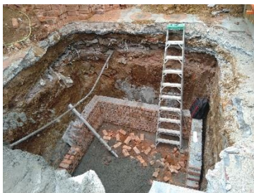
Day 4 Settling tank brickwork started
