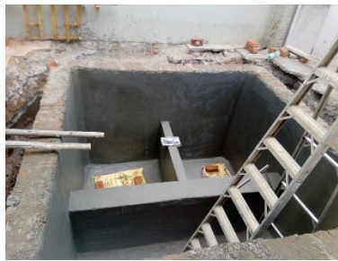
Day 11 Plastering of bio-chamber and other internal walls
