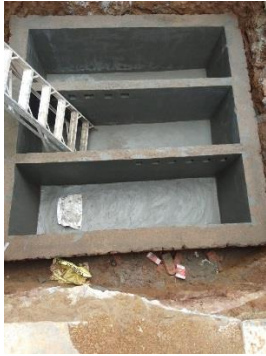
Day 7 Settling tank plastering and bed completed
