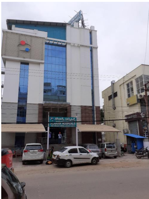
Konark Hospitals. Blue shed on the right houses the STP filters.
