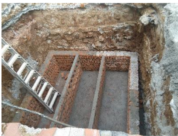
Day 5 Settling tank brickwork completed with dividers
