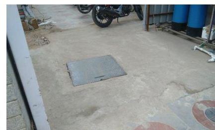
Day 15 Finishing touches and setting of manhole lids.
