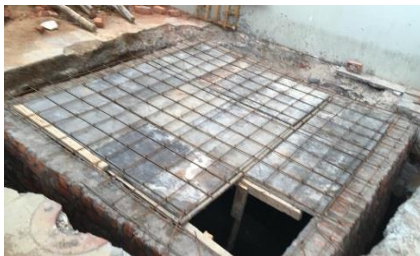
Day 12 Top slab centering
