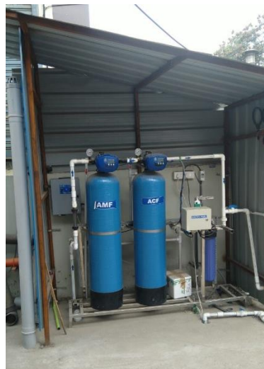
Original WTP setup with AMF, ACF, bag filter and UF. Current WTP setup with ozonator, bag filter, AMF, ACF and MCF.
