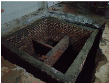
Day 10 Bio-chamber walls constructed
