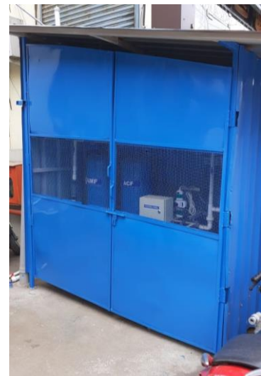
Original WTP setup with AMF, ACF, bag filter and UF. Current WTP setup with ozonator, bag filter, AMF, ACF and MCF.
