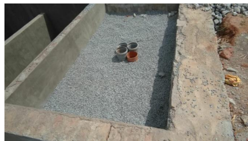
Settling tank, reed-bed, two hummus tanks (waiting to be covered) and percolation pit.
