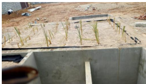
Settling tank, reed-bed, two hummus tanks (waiting to be covered) and percolation pit.
