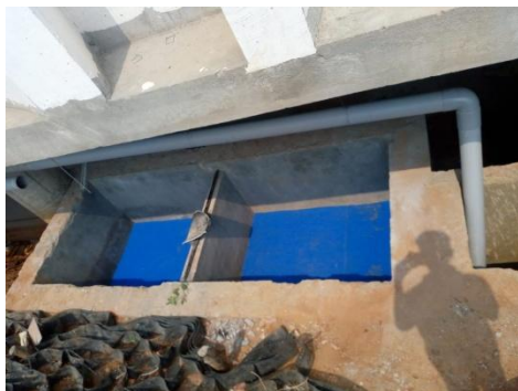
Bio-chamber with mats and center rod in place. Protective structure for Aquatron® being built.
