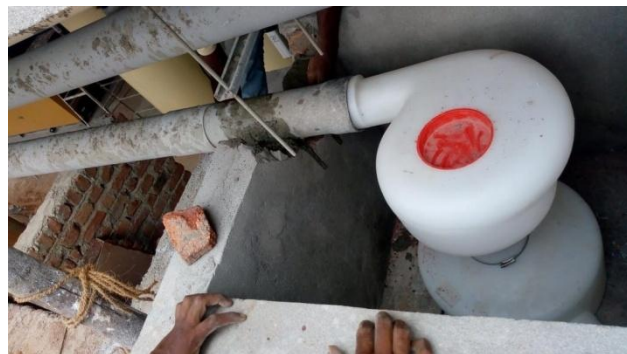
Bio-chamber with mats and center rod in place. Protective structure for Aquatron® being built.
