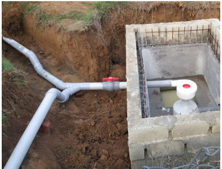
Sacred Grove Ashram, Madanapalle Pipes from multiple buildings connected to one Aquatron
