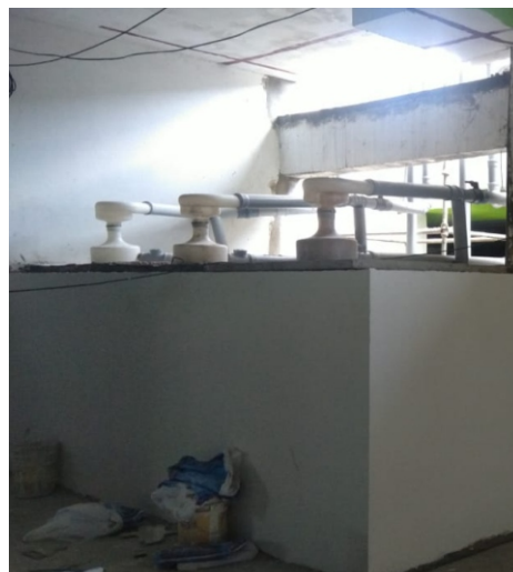
Sandhya Elite IT tower, Hyderabad Bio-chambers in basement dead spaces
